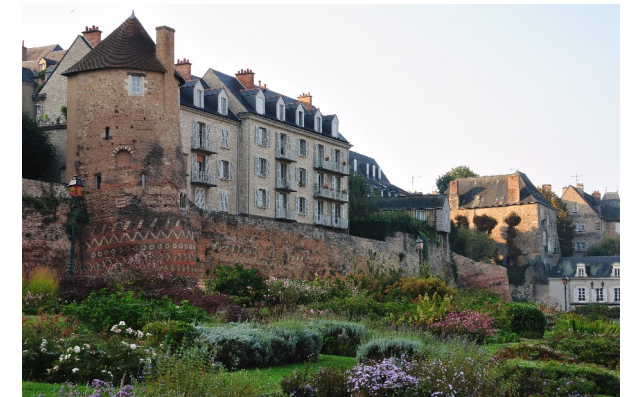
The ramparts, Gallo-Roman wall.
